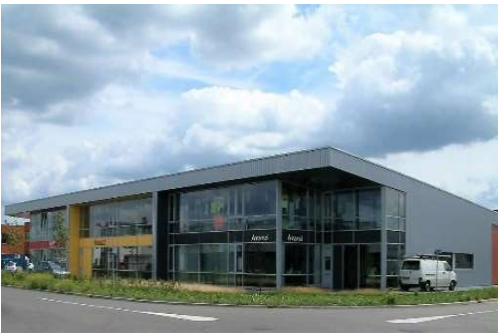
SEK Building Paxtonstraat 23, 25, 27.
